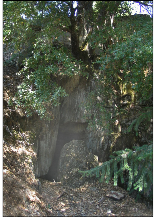
Figure 17. Tunnel beneath the right road abutment at Steephollow Crossing was the spillway for a dam at this site from 1924 to 1925.
